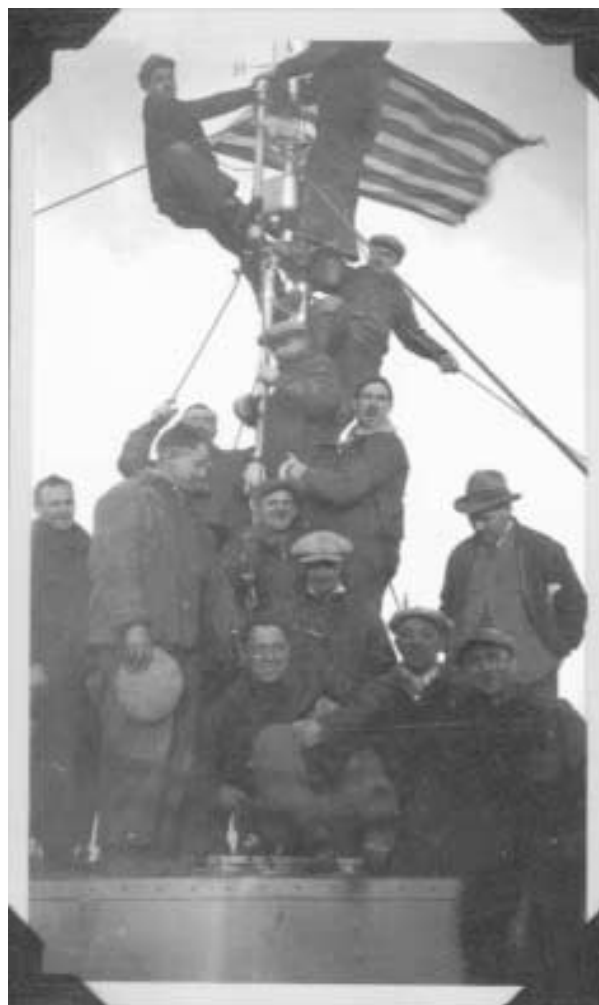
Workers raise the topping out flag on the completed mooring mast of the Empire State Building (March 18, 1931).
